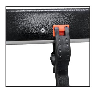
Measure 1  $\frac{1}{2}$ " from the back of the track and up  $\frac{1}{2}$ " from the bottom of the top and mark the rear hole for the track. Use the  $\frac{1}{8}$ " drill bit to drill the mounting hole and install the pop rivet.
